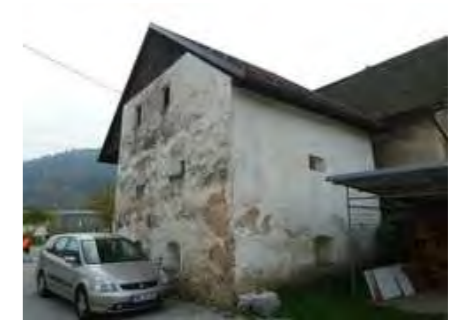
Pogled na S in Z fasado
